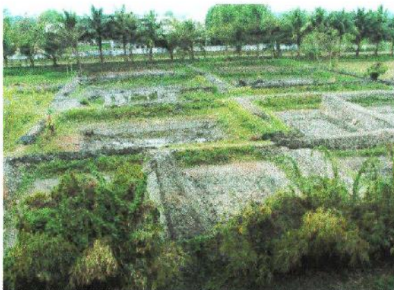
Experimental pond after digging and dike preparing
