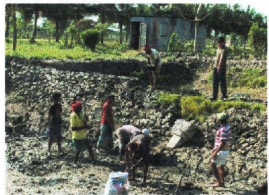
Experimental pond during bottom mud removing, digging and dike repairing
