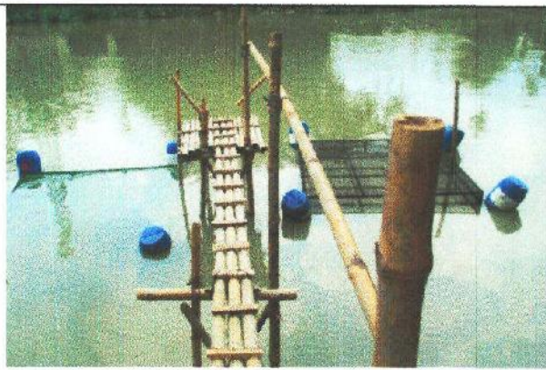
Fig 7: One of the cages was damaged due to high tide and strong current
